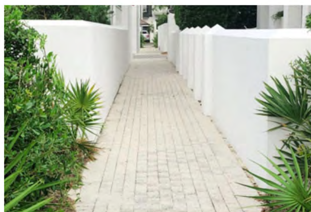
columns with a point
