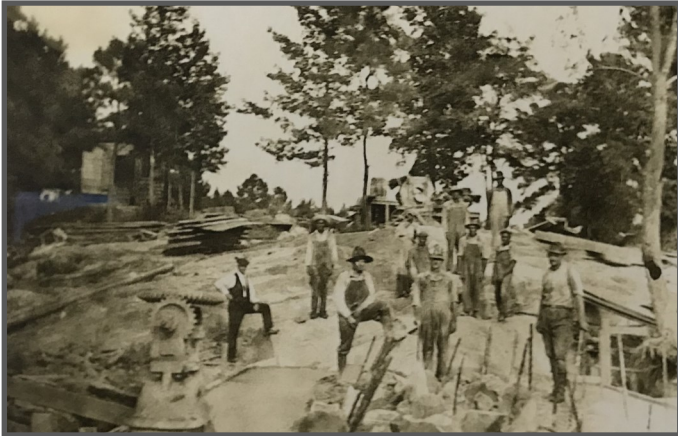
Photos: Various perspectives of dam being rebuilt
