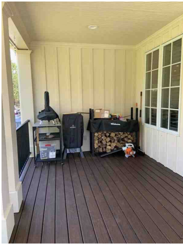
Rear Covered Porch
