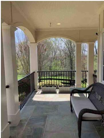
Covered Front Porch View 3
