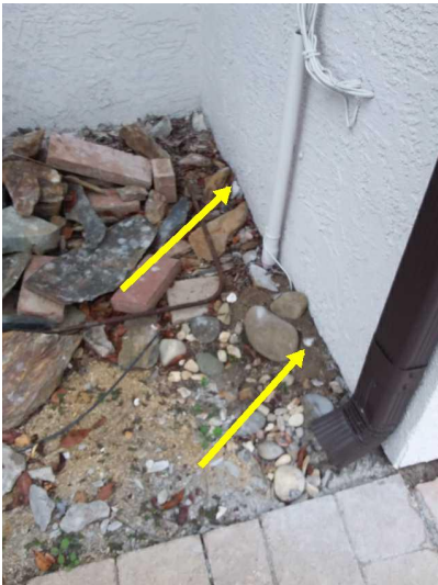
The soil is too high against the home at various areas around the home which should serviced.
