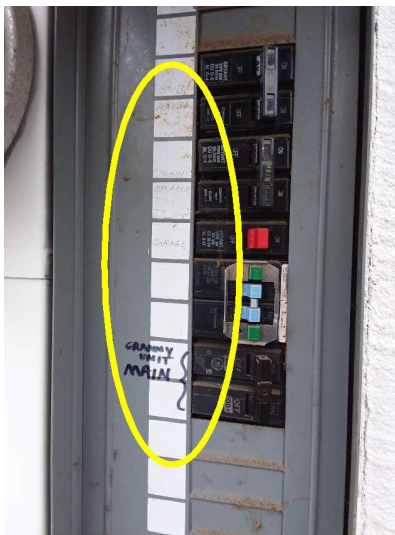
Various circuits are not labeled, which is recommended.
