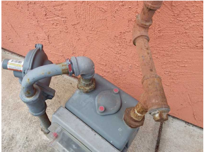
Some of the gas lines at the meter are rusted and should be painted to prevent further corrosion.
