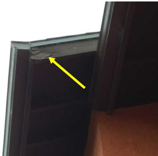
There is moisture damage or dry rot to the wood trim and or fascia on the upper roof area, which is typically not inspected by the pest inspector. The pest control company should be alerted so as to inspect and include these repairs in their estimate.
