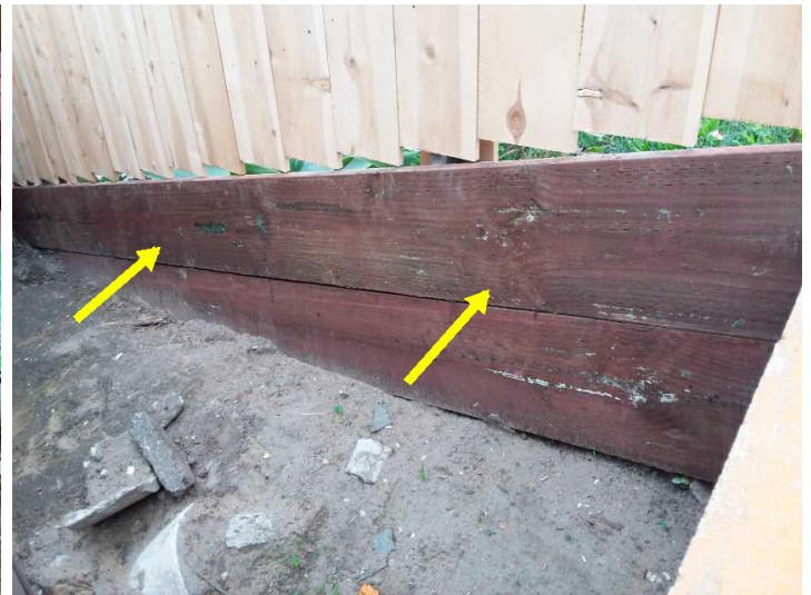
The wooden planks at the rear of the property have no structural value, and are intended to inhibit surface soil movement, and should be periodically monitored for damage or stability.
