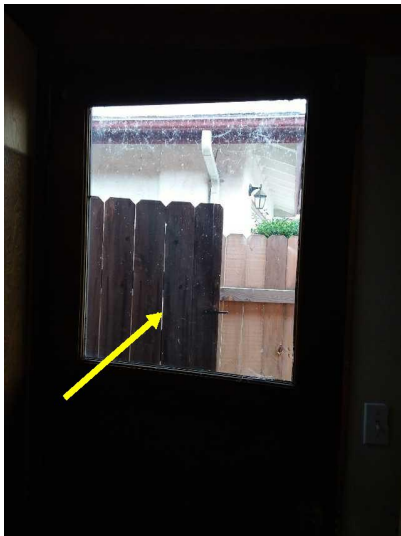
The window panes are not tempered or safety glass which is required by current standards.
