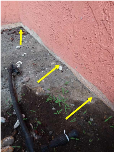
The soil is too high against the home at various areas around the home which should be serviced.
