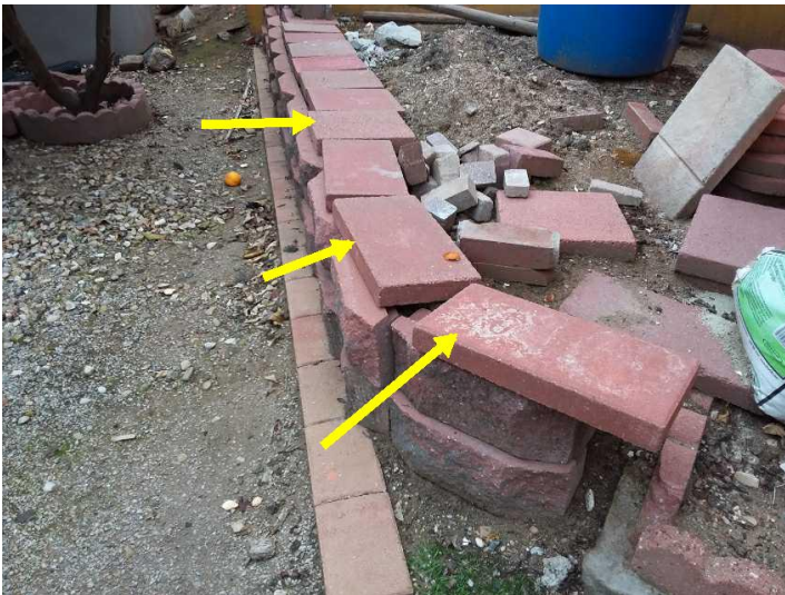
Some of the planter block-caps are loose or missing and should be serviced.
