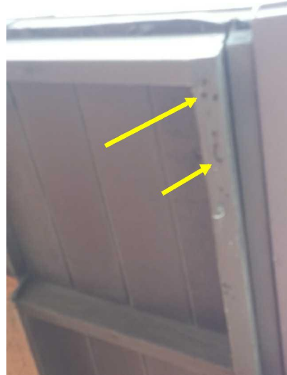
There is damage to the wood trim that should be evaluated by a termite inspector.
