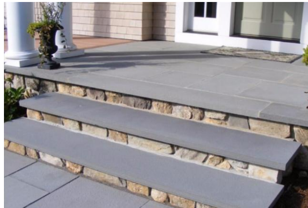
FRONT STEPS: BLUESTONE SLAB & STEPS
