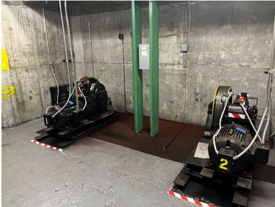
15. View of the elevator motors.
