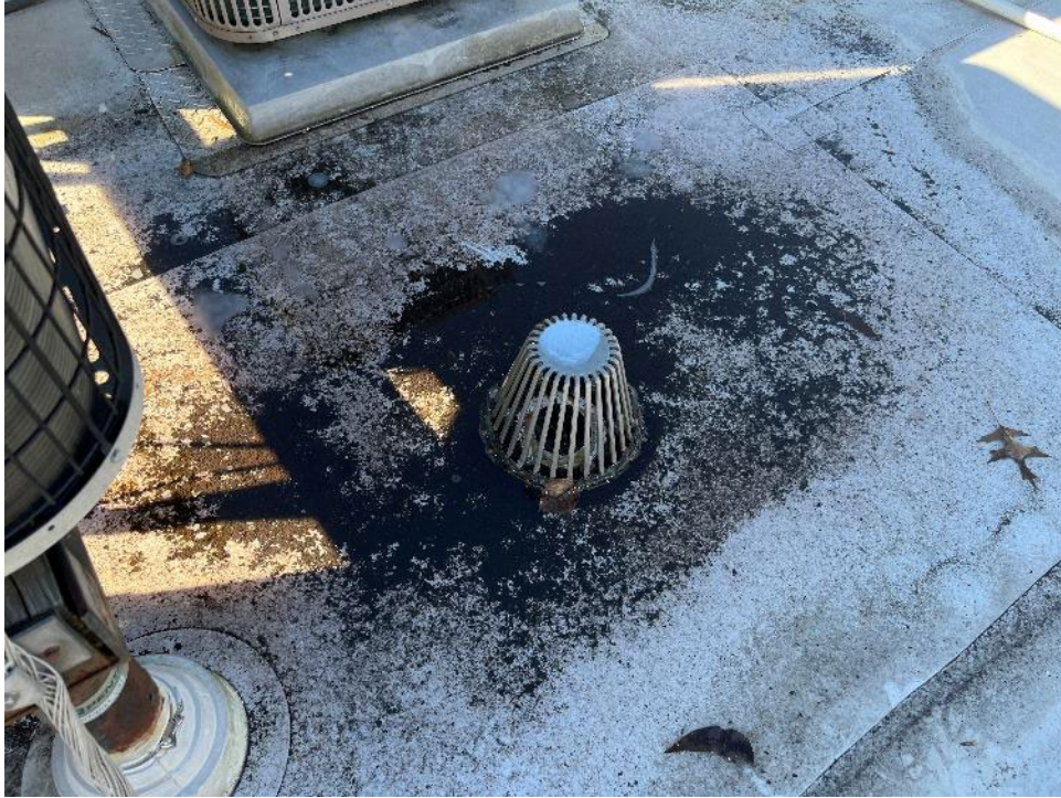
7. View of accumulated debris around roof drains.
