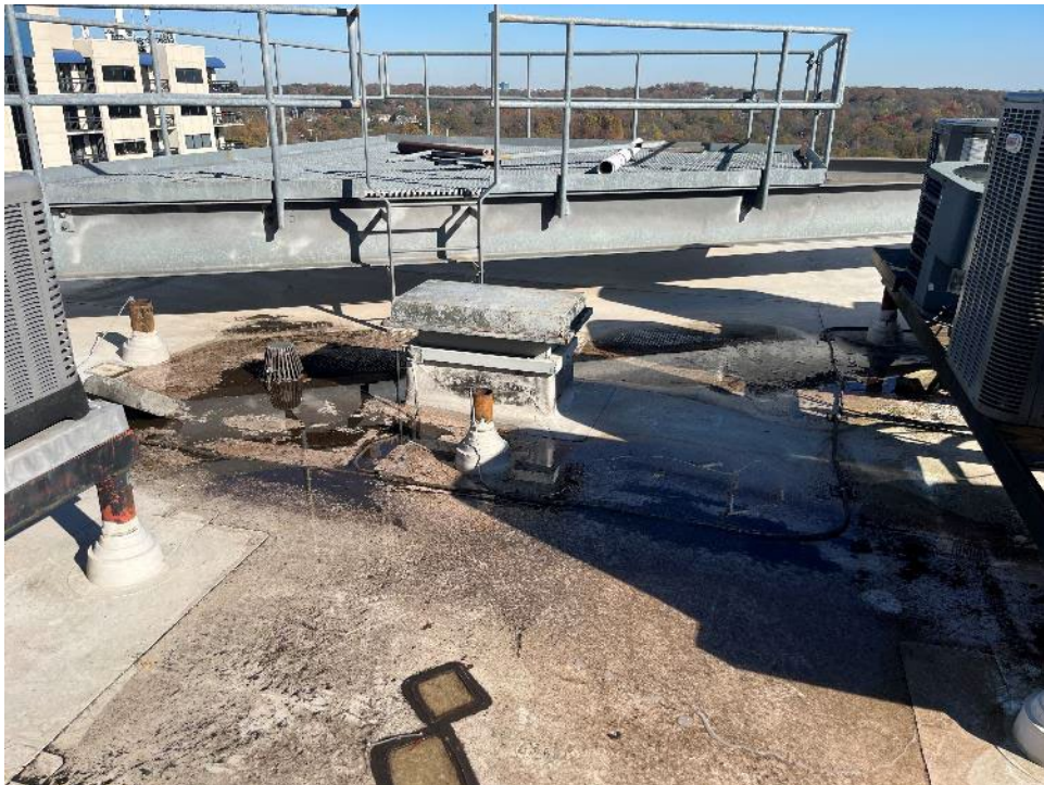
8. View of ponding water at one of the roof drains.
