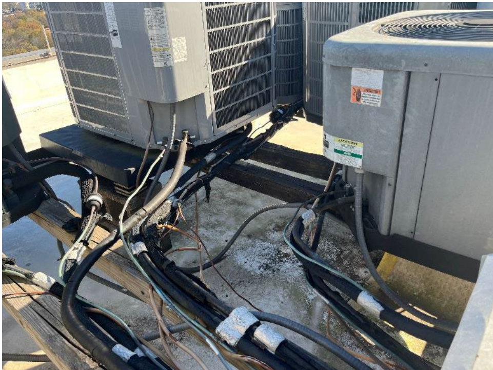
10. View of deteriorated and deflected HVAC supports.
