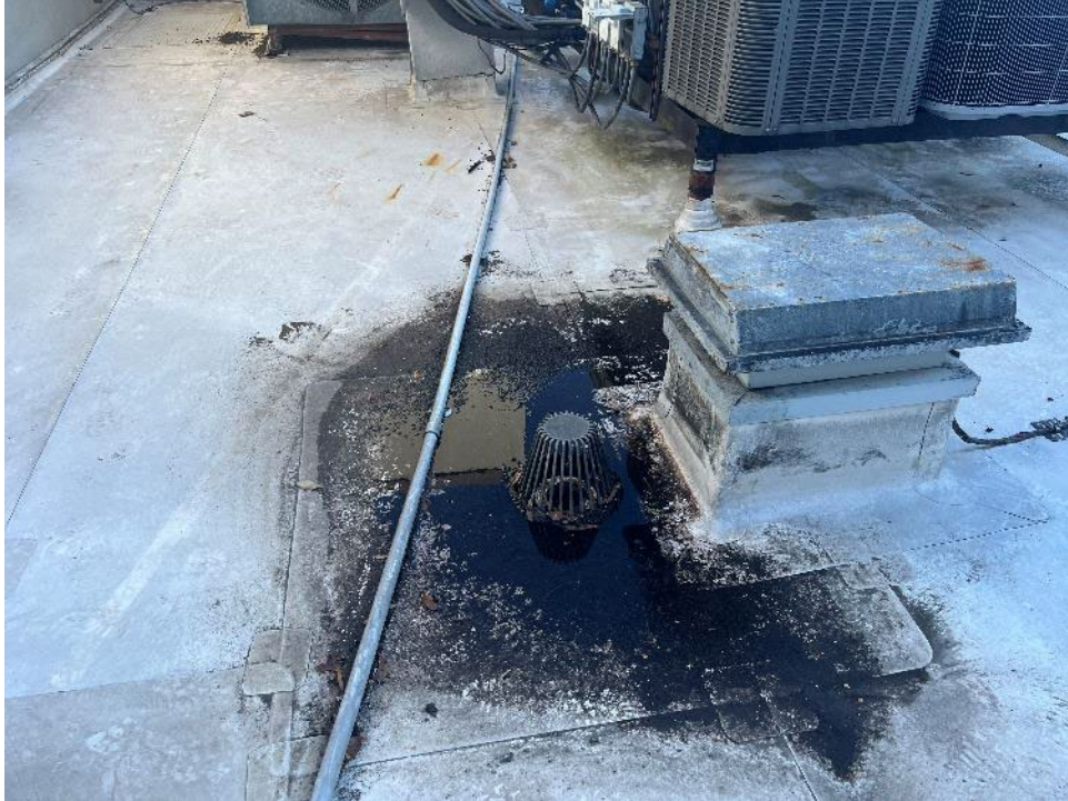
9. View of ponding water and accumulated debris at a roof drain.
