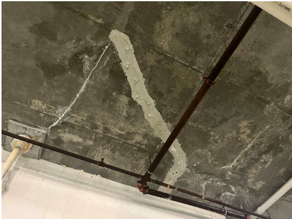
14. View of hairline cracks in the ceiling of the parking garage that were previously sealed.
