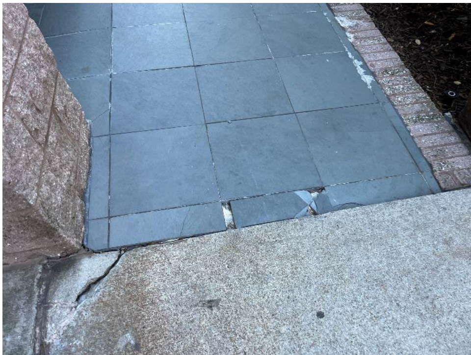
2. View of cracked tiles near the building entry.
