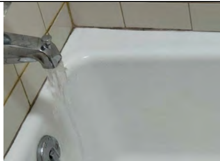
Diverter Did Not Function Properly
