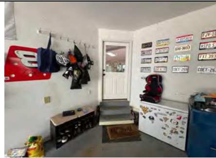
Non Fire-Rated Garage Service Door
