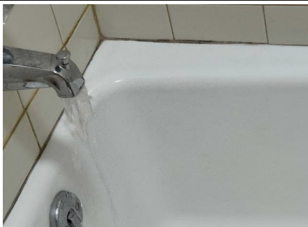
Diverter Did Not Function Properly
