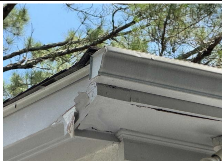
Damaged/Deteriorated Trim & Soffit
