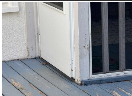
Damaged/Deteriorated Trim
