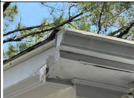
Damaged/Deteriorated Trim & Soffit
