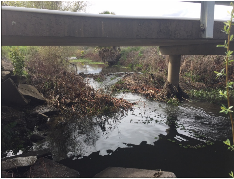
Existing pedestrian bridge, looking upstream. One of 2 concrete center support columns that will be removed is visible. Concrete rubble in the bed and along banks of the creek, (foreground) will also be removed to accommodate terrace construction.
