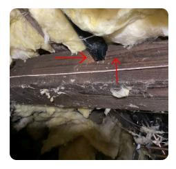
85 Deteriorated Rafter And Framing
