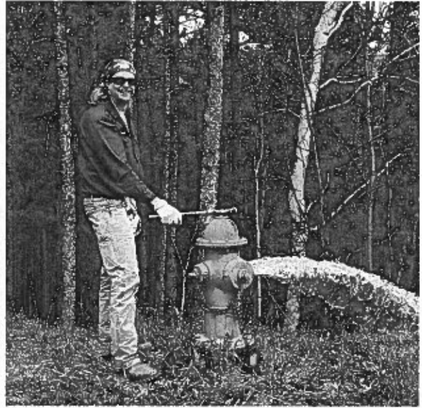
Utilities staff performing annual maintenance on a fire hydrant.
