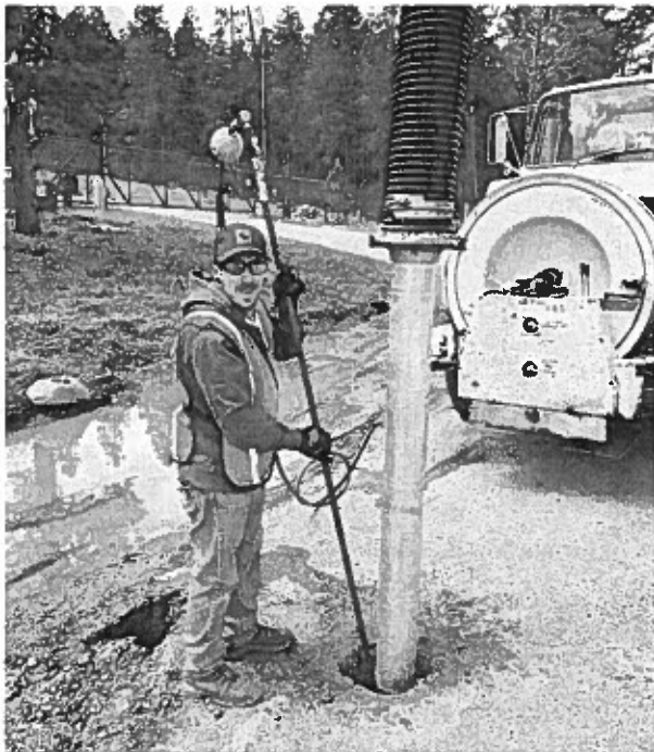
Utilities staff locating underground infrastructure.
