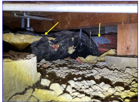
Damaged/missing insulation
