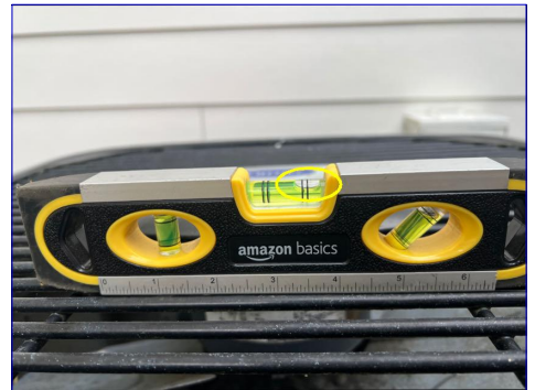
Unit is out of level
