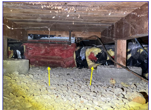
Damaged insulation
