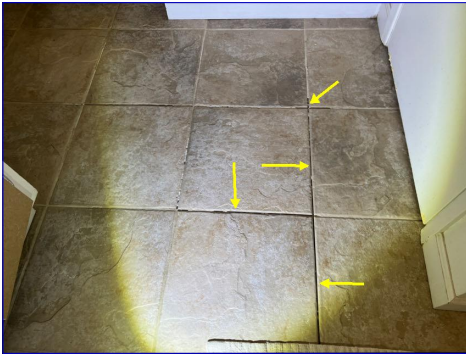
Deteriorated grout
