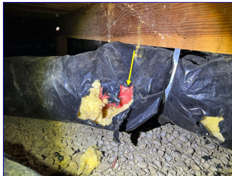
Damaged insulation
