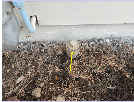
Sewer line clean out
