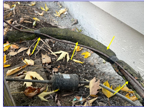
Missing/weathered insulation
