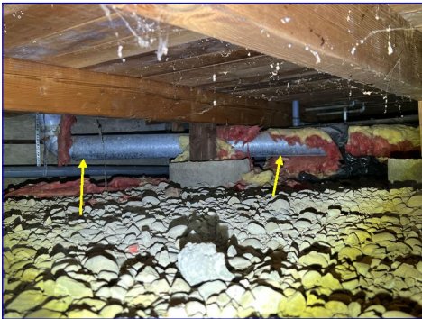
Damaged/missing insulation
