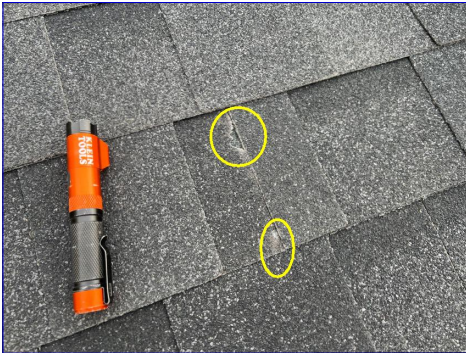
Damaged/chipped shingle
