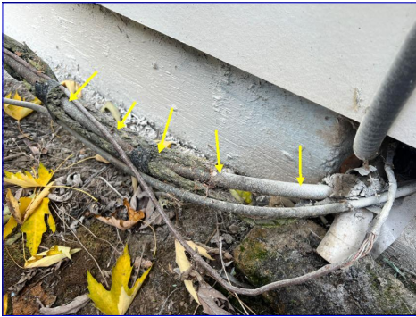
Missing/weathered insulation
