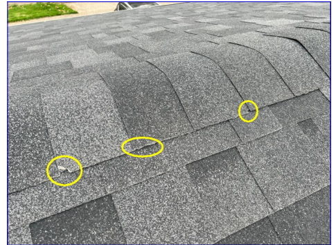
Damaged/chipped shingles
