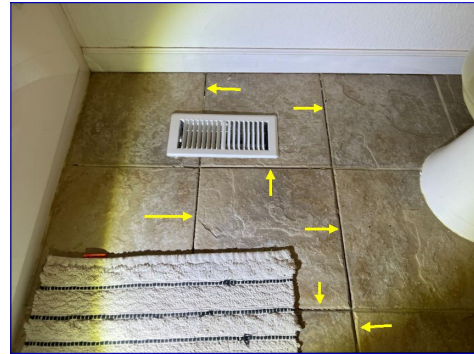
Deteriorated grout
