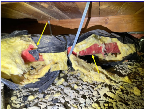
Damaged insulation
