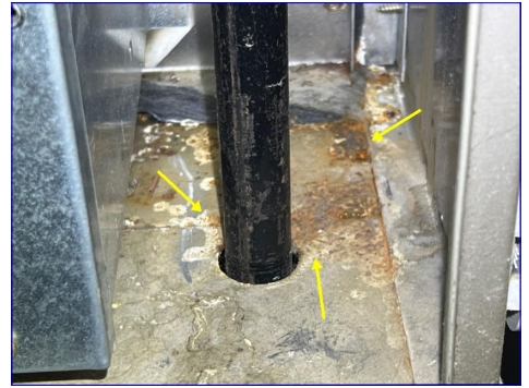
Rust/corrosion
