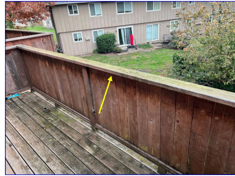
Loose guardrail
