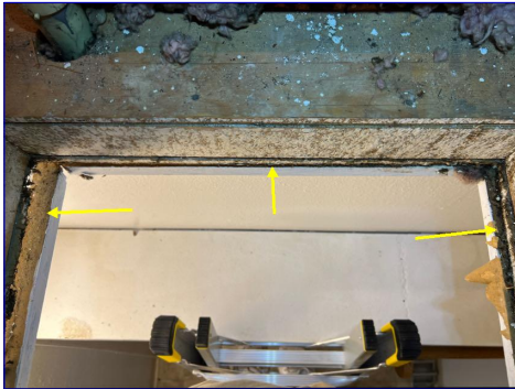
Missing weatherstripping
