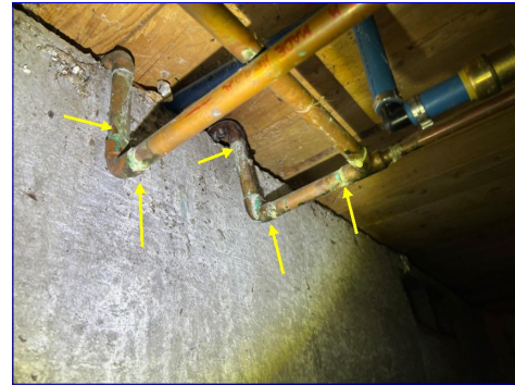
Minor corrosion
