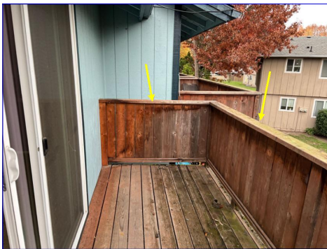
Loose guardrail
