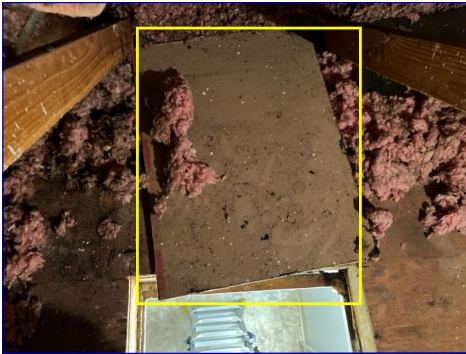
Missing insulation
