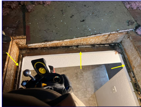
Missing weatherstripping
