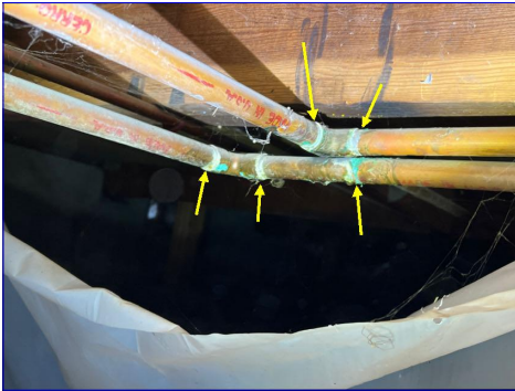
Minor corrosion
