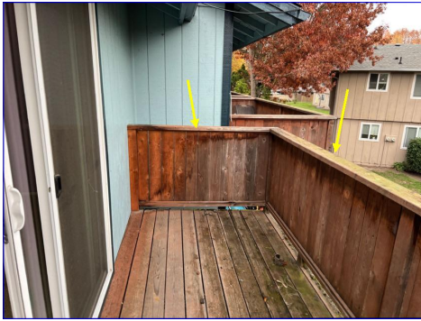
Loose guardrail
