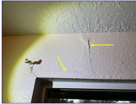
Common crack
