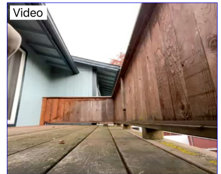
Loose guardrail
