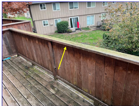
Loose guardrail
