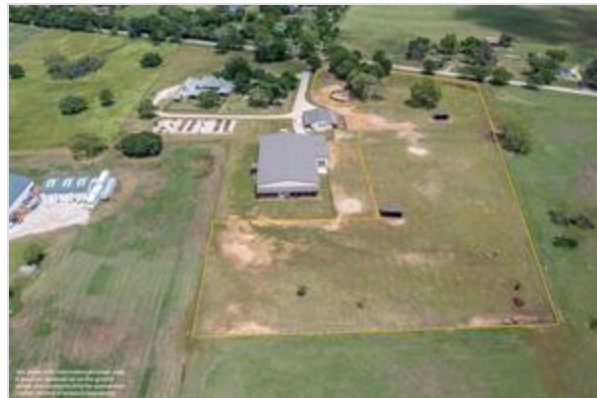
Overhead View facing North
