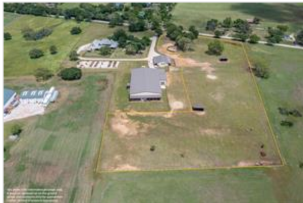
Overhead View facing North
