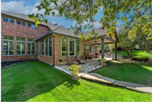
BACK OF HOME AND PATIO
