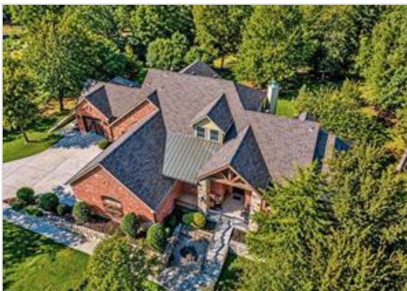
FRONT OF HOME...Aerial View
