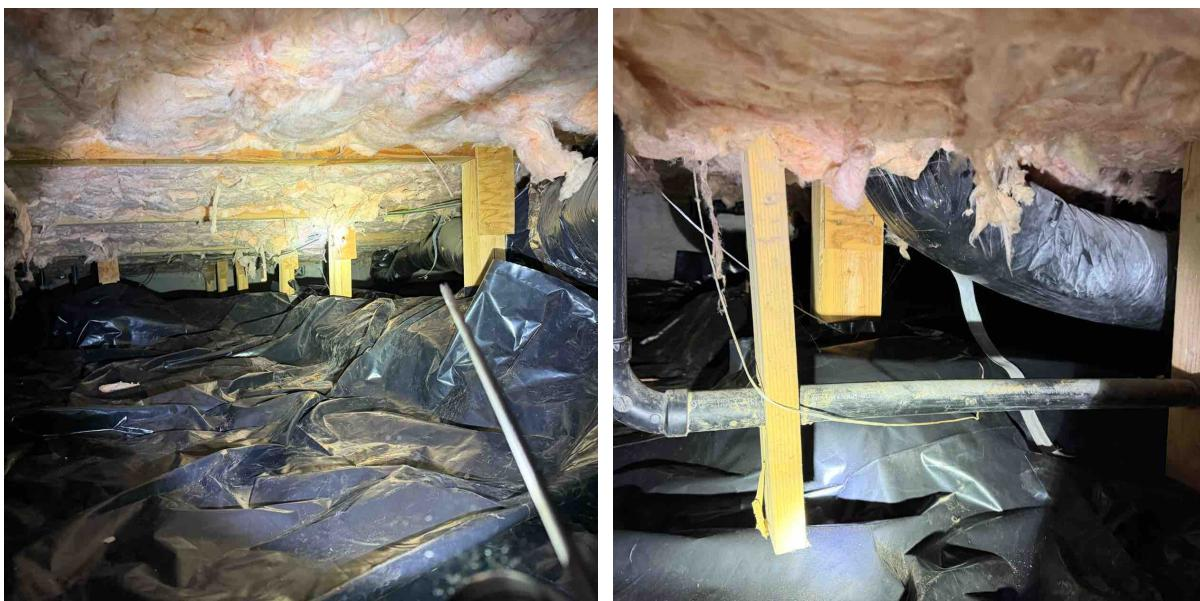
6.1.3 The crawlspace has been largely updated with 6mill black visqueen throughout, and newer, fiberglass insulation.
