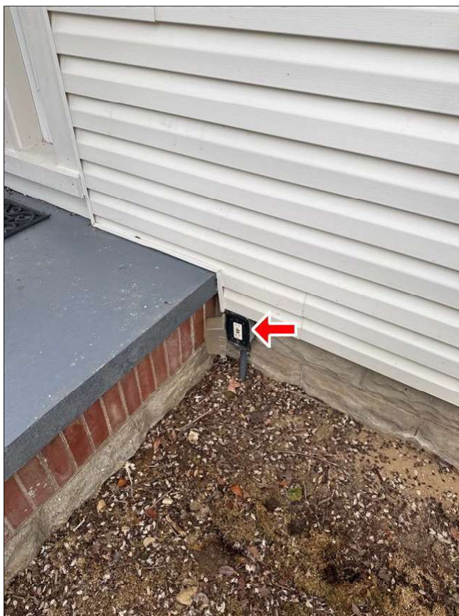
5.7 Item 1(Picture) Receptacle would not reset, was not functional
