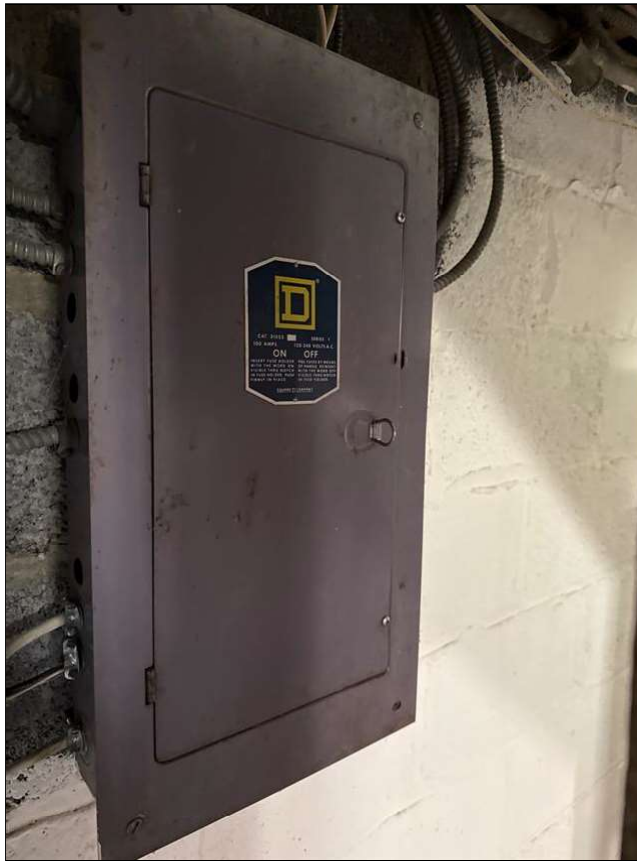
Former panel, serving as a sealed junction box
