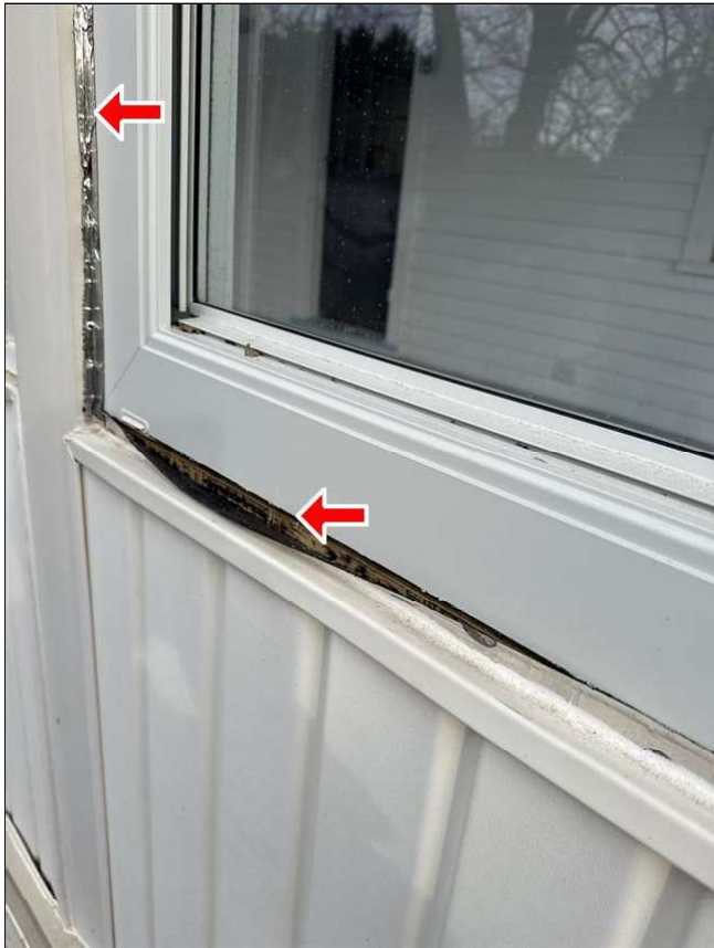
2.0 Item 1(Picture) Exposed flashing tape, not rated for exposure
