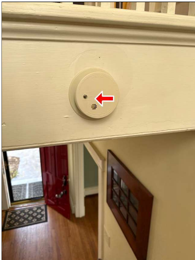
5.9 Item 1(Picture) Smoke alarm was not functional
