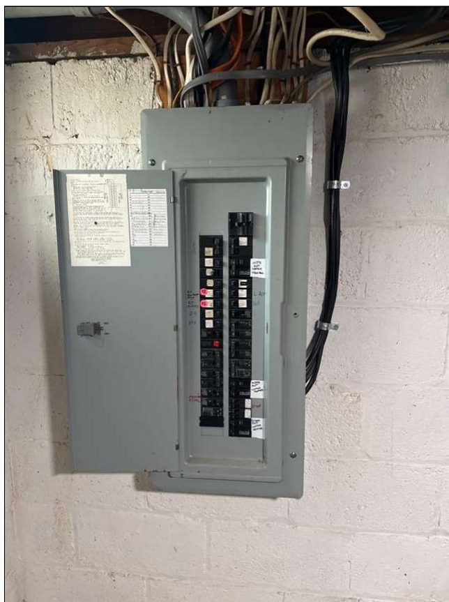
Service panel and main disconnect
