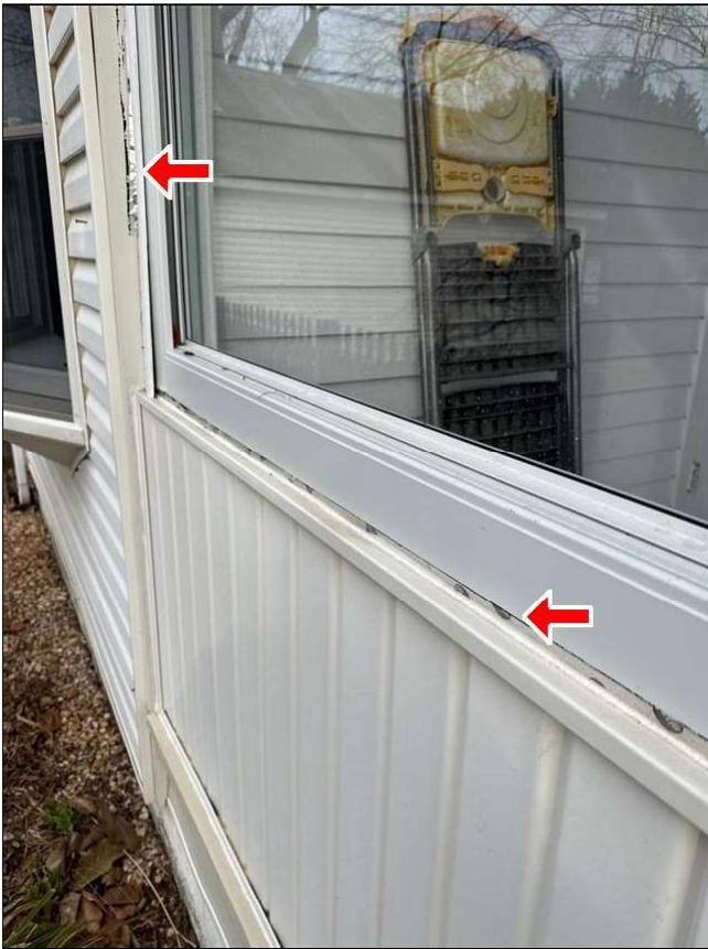
2.0 Item 3(Picture) Exposed flashing tape, not rated for exposure
