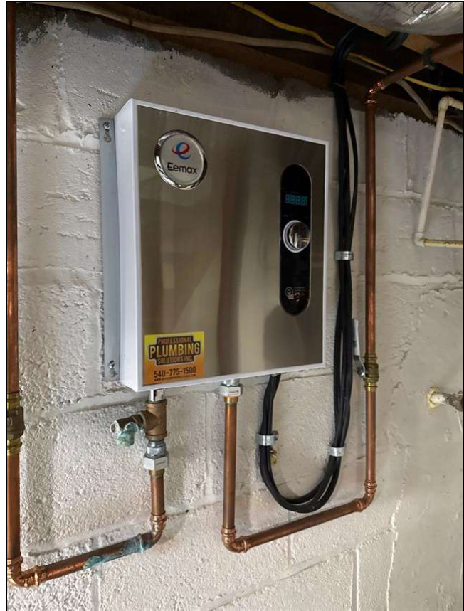
Electric tankless water heater
