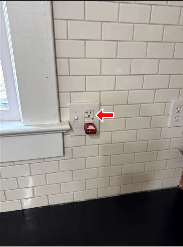
5.7 Item 3(Picture) Receptacle would not reset, was not functional
