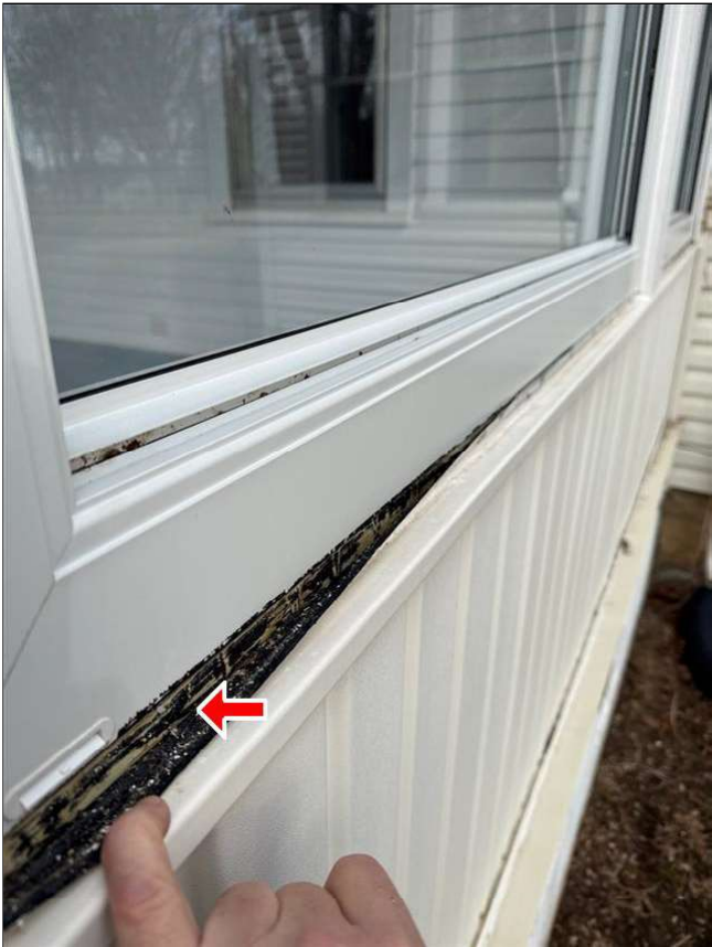
2.0 Item 2(Picture) Flashing tape, peeling away from wall sheathing
