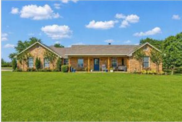
FRONT OF HOME...Close View
