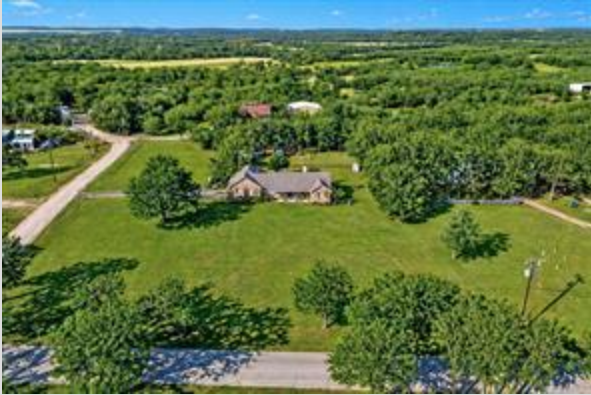
FRONT OF PROPERTY...Aerial View
