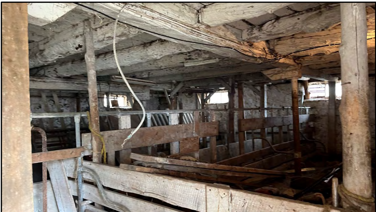
Photo 10 | View Inside Bank Barn – First Floor | Looking Northwest
