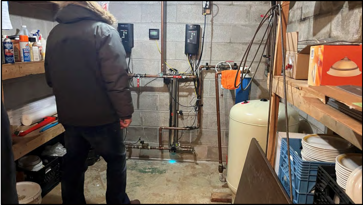
Photo 25 | View of Water Room in Basement Addition
