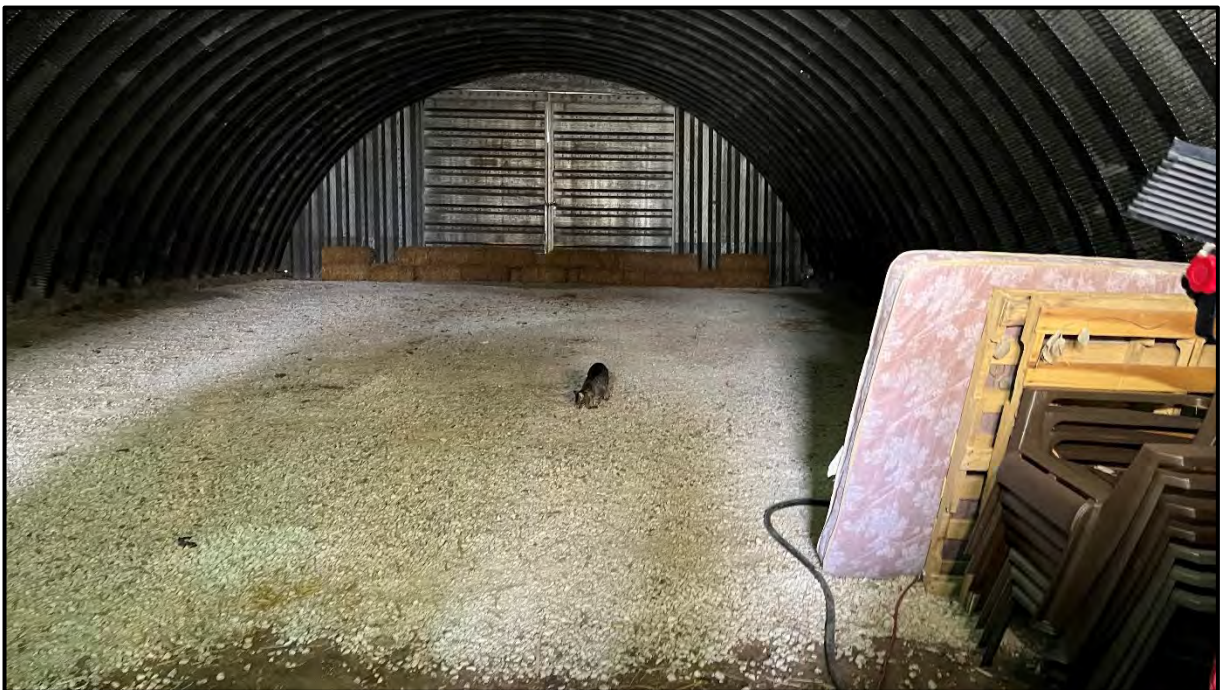
Photo 6 | View Inside Quonset Hut | Looking South
