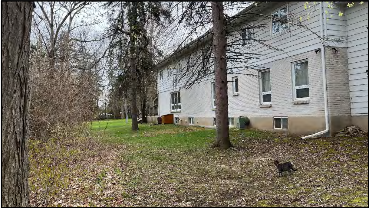
Photo 3 | View of East Property Boundary and Addition | Looking South
