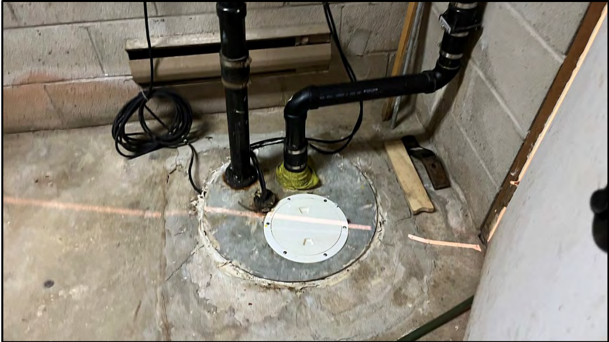
Photo 27 | View of Sludge Pit in Basement Addition
