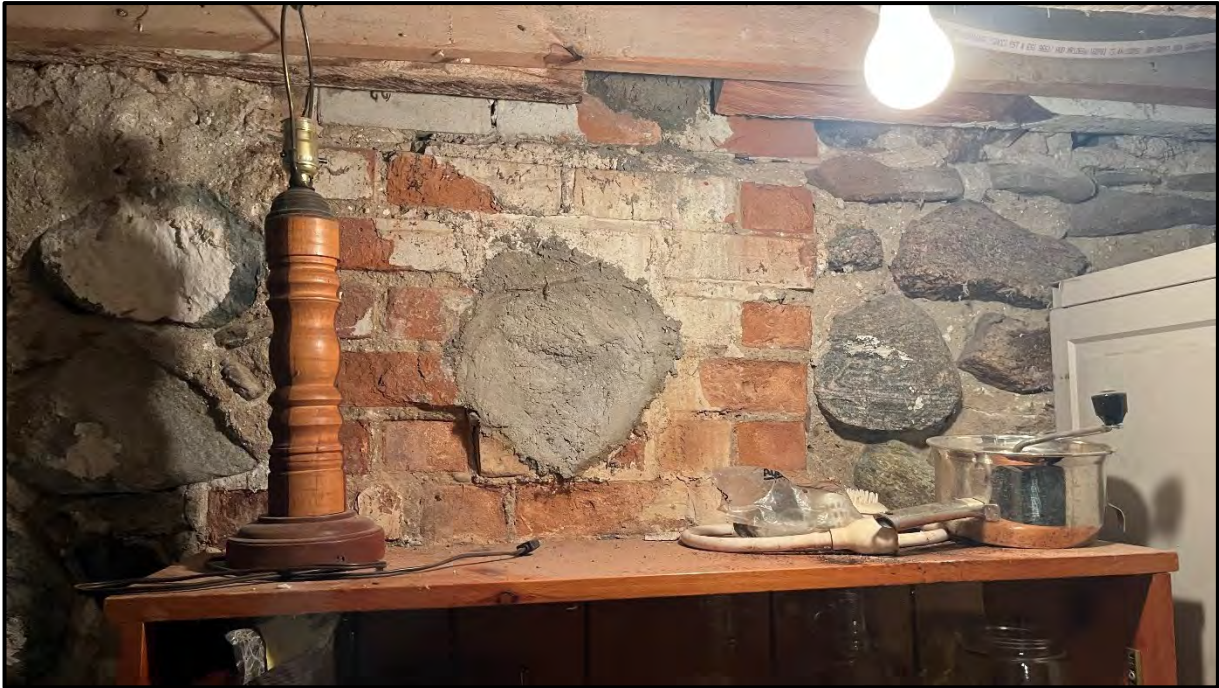
Photo 19 | Former Chimney In Original Basement
