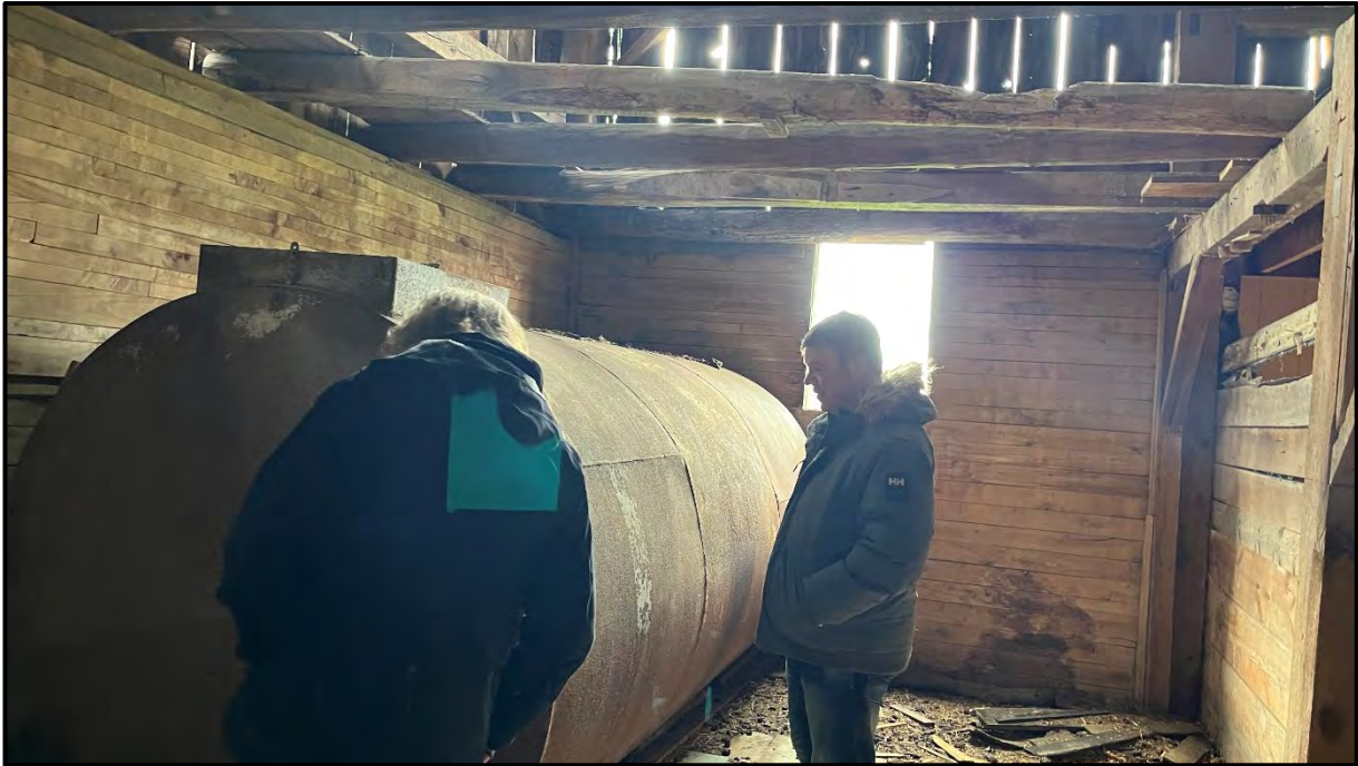
Photo 11 | View of AST Used to Collect Rain Water – 2 nd Floor of Bank Barn | Looking South
