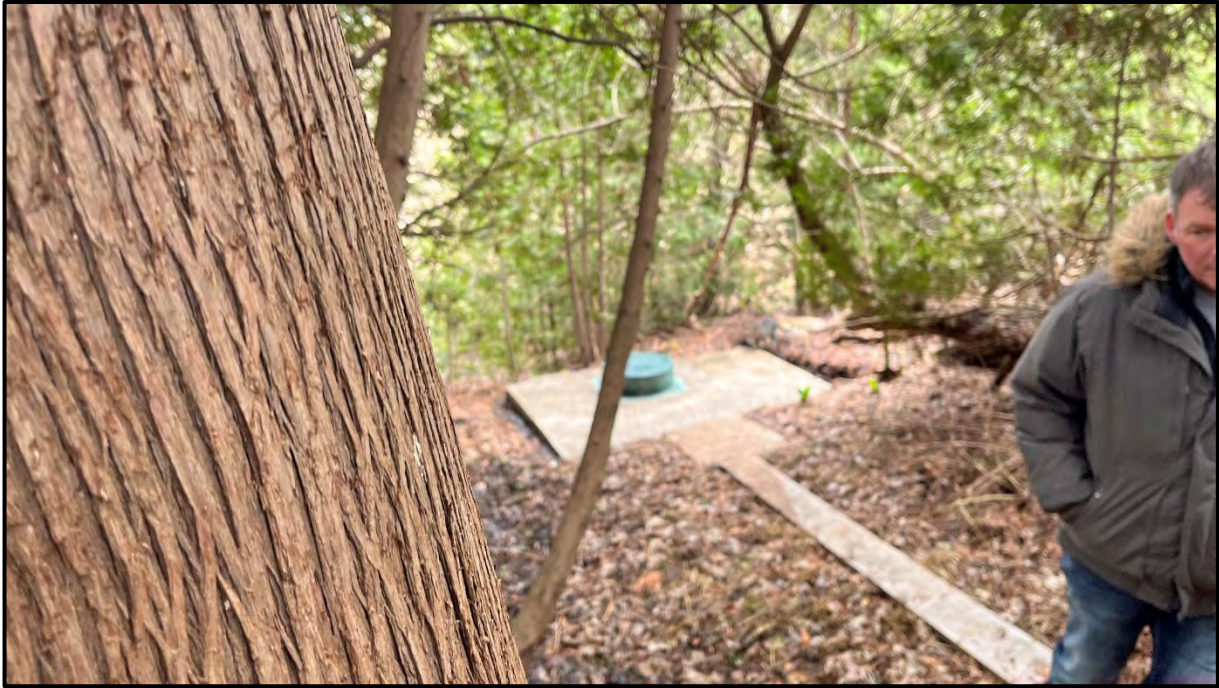
Photo 13 | View of Drinking Water Cistern | Looking East
