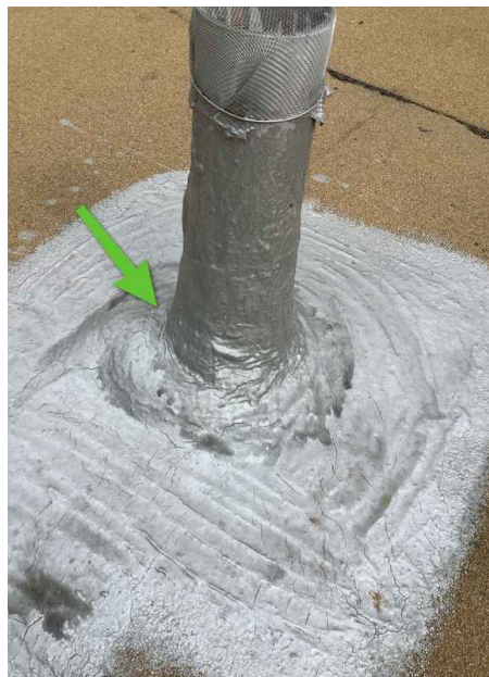
example of roof penetrations
