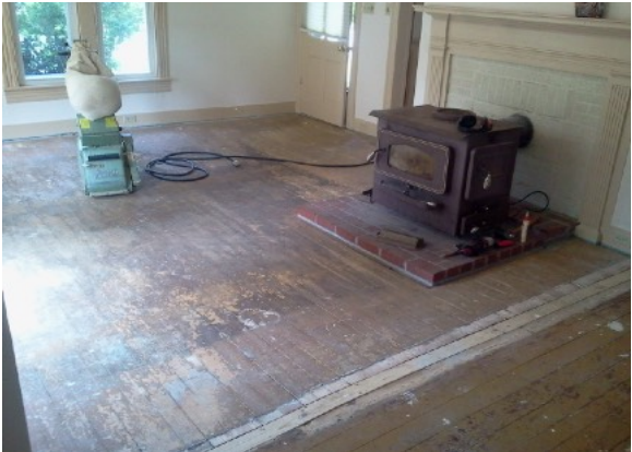
Figure 8: Living room floor prepared for sanding
