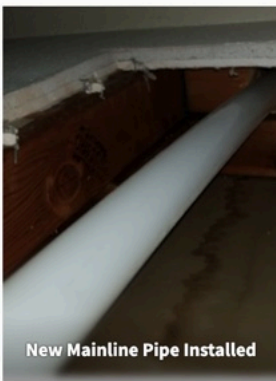
Lead Toilet Drain Pipes- ABS Replaced
