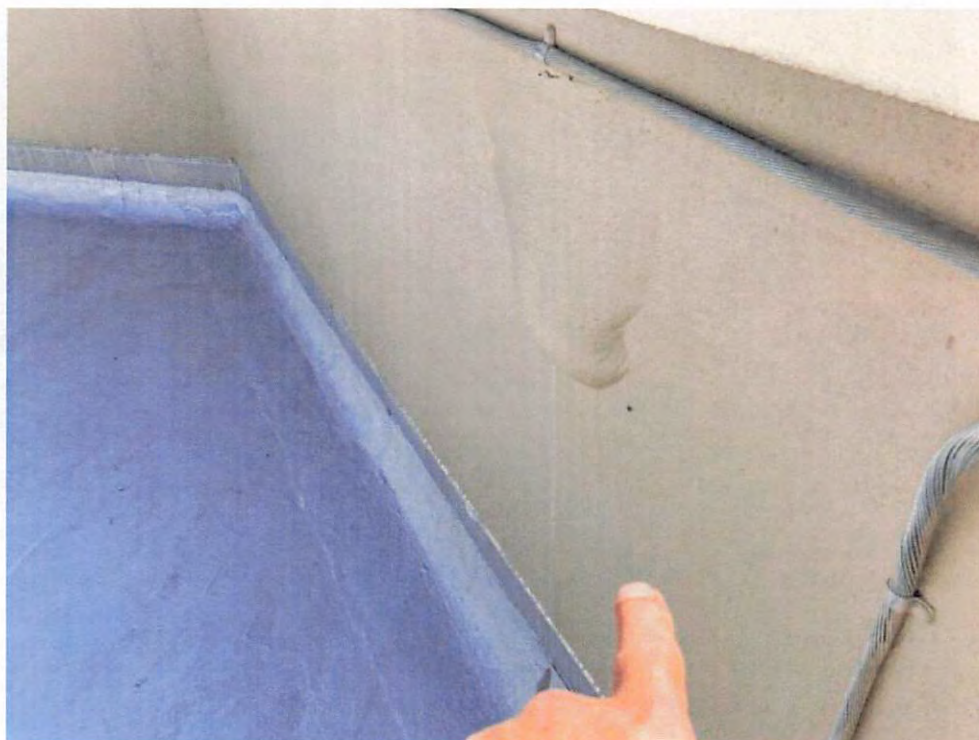
Figure 8 – Roof Parapet Wall.
