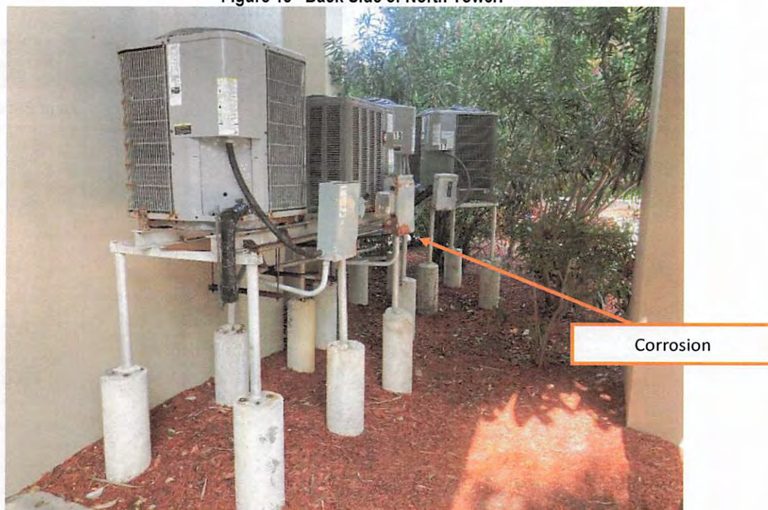
Figure 16 - South Tower A/C Equipment.
