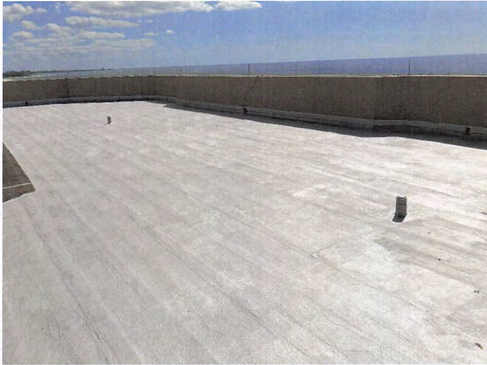
Figure 1 – North Tower Roof Deck
