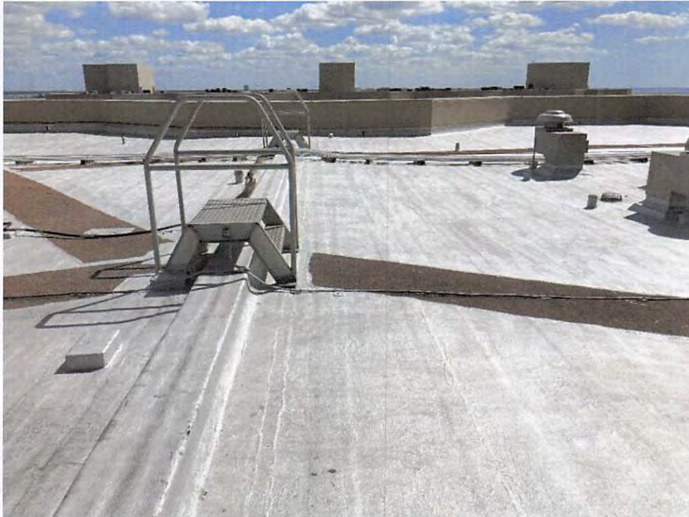
Figure 1 - South Tower Roof Deck
