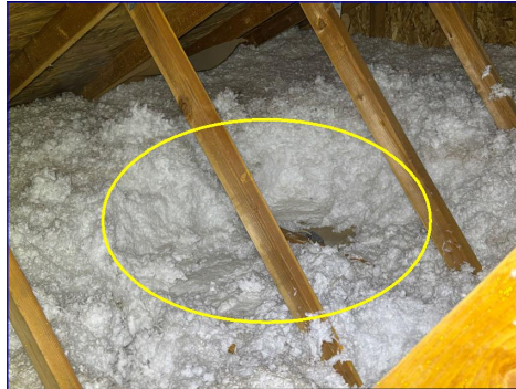
Disturbed insulation
