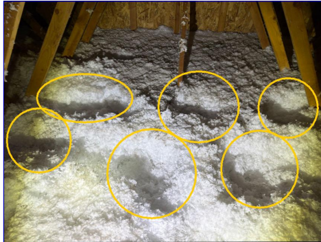
Disturbed insulation
