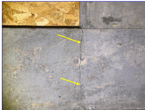
Foundation crack
