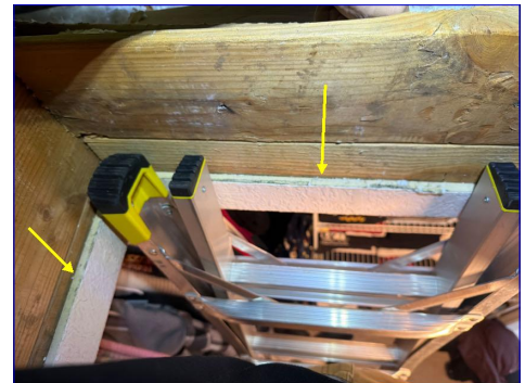
Missing weatherstripping
