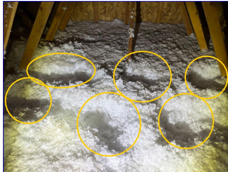
Disturbed insulation
