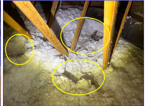
Disturbed insulation
