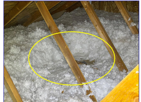
Disturbed insulation
