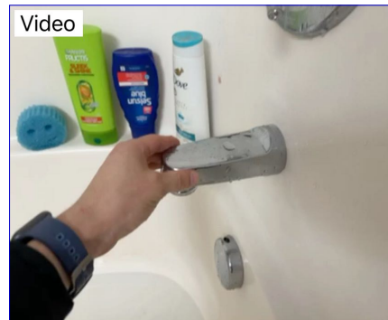
Loose tub faucet
