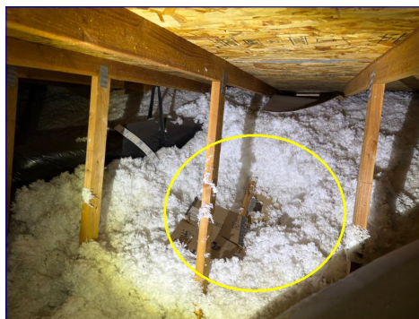
Disturbed insulation
