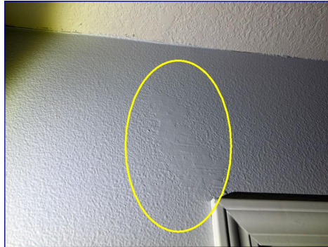
Patched crack
