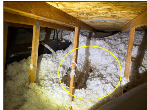
Disturbed insulation
