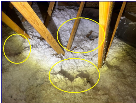
Disturbed insulation
