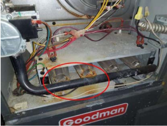
Photo 6: Service Heat/Maintance Lacking.
