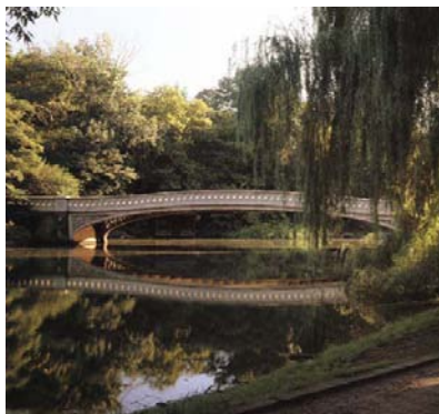
Photo showing the Bow bridge at Central Park
