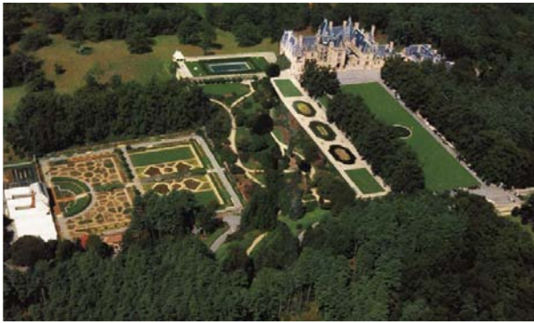
Aerial view of the Biltmore Estate®
