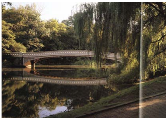
Photo showing the Bow bridge at Central Park
