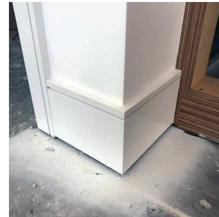
Painted base moulding and door casing detail
