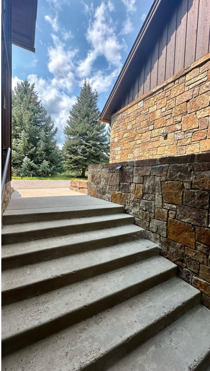
Garden Level Exterior Stairs
