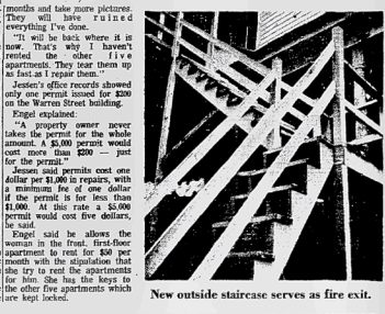
New outside staircase serves as fire exit.
