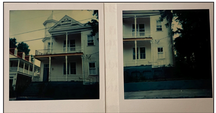
Figure 9: 1980 photographs showing porch repairs (City of Charleston Board of Architectural Review)
