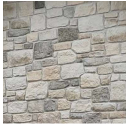
Exterior Stone Mortar Application White Over grout
