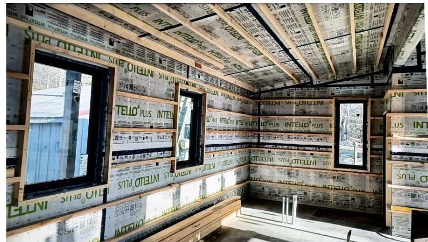
Installation reference showing membrane continuity before interior finishes.
