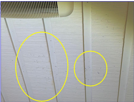
Possible microbial growth (Primary bathroom)
