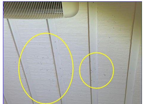
Possible microbial growth (Primary bathroom)
