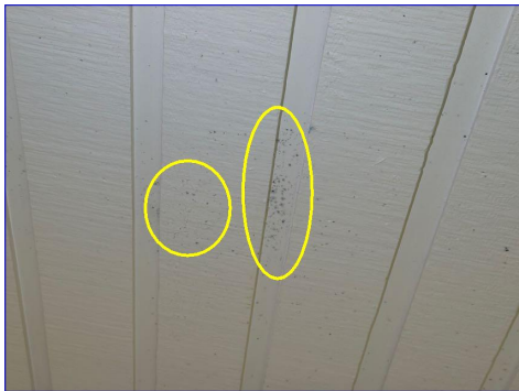
Possible microbial growth (Primary bathroom)
