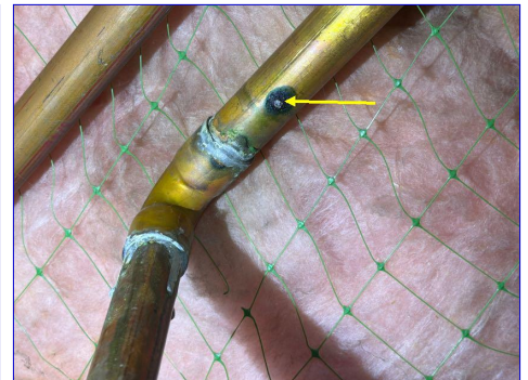
Minor corrosion
