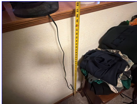
Window sill exceeds 44"
