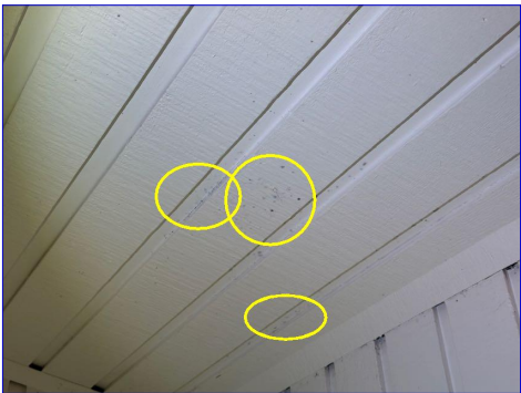
Possible microbial growth (Primary bathroom)
