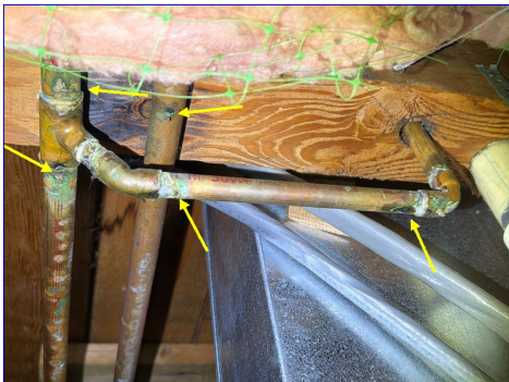
Minor corrosion
