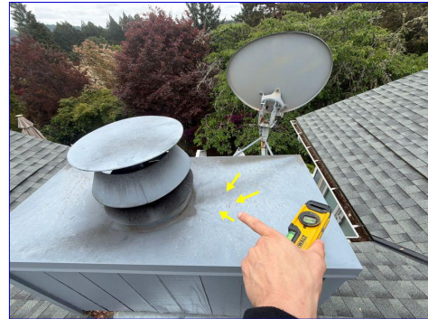
Negative slope (south side)
