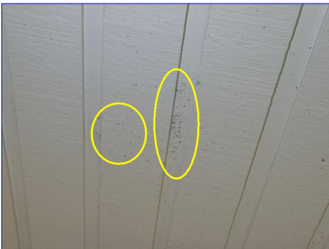
Possible microbial growth (Primary bathroom)
