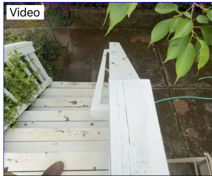
Loose handrail
