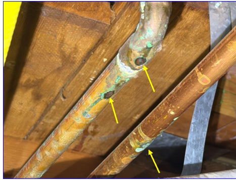
Minor corrosion
