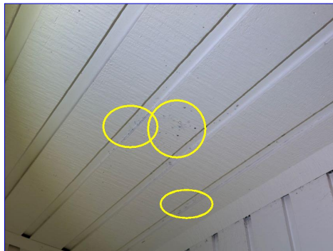
Possible microbial growth (Primary bathroom)
