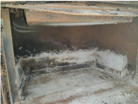
Photo 45: Inspect/Clean Fireplace Chimney.
