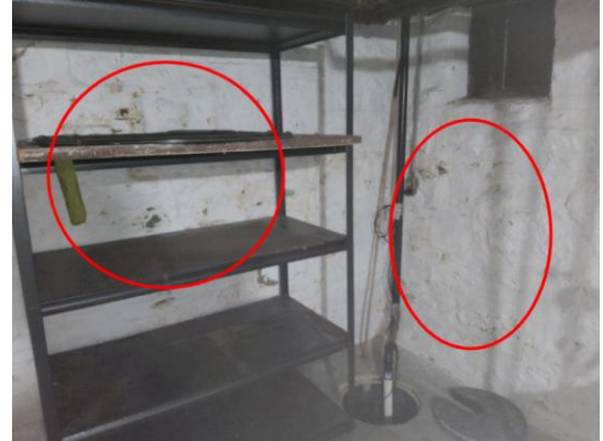
Photo 2: Surface Deterioration.
