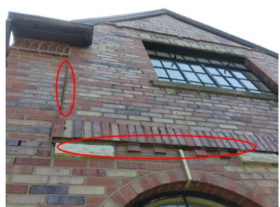
Photo 4: Cracks Moderate.
