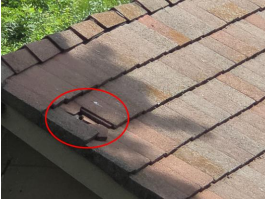
Photo 5: Missing/Damaged Shingles.
