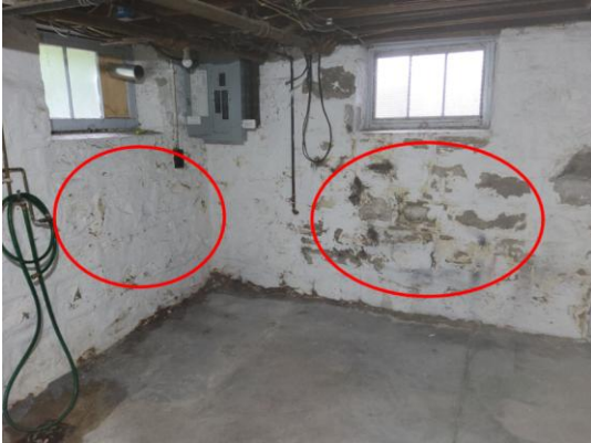
Photo 1: Surface Deterioration.
