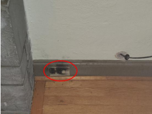
Photo 23: Overheated Outlets.
