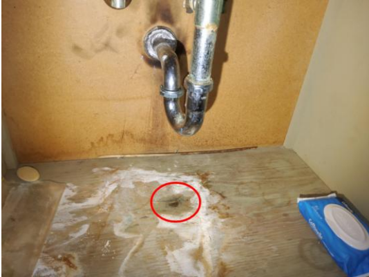
Photo 29: Pipe Leak.
