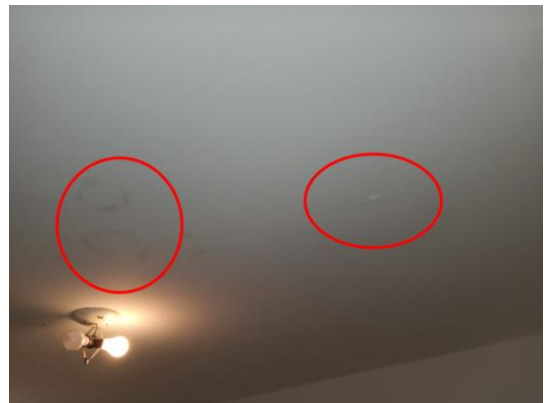
Photo 37: Water Damage.
