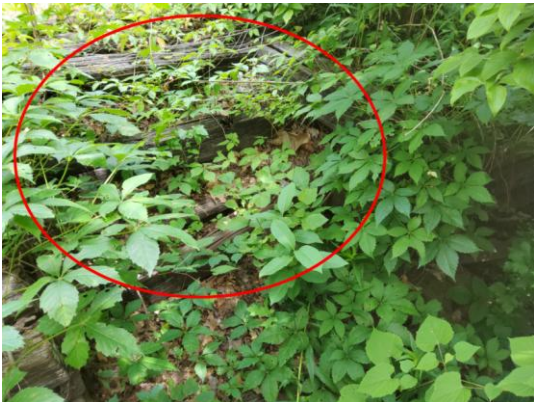
Photo 16: Wood Stairs Dilapidated .
