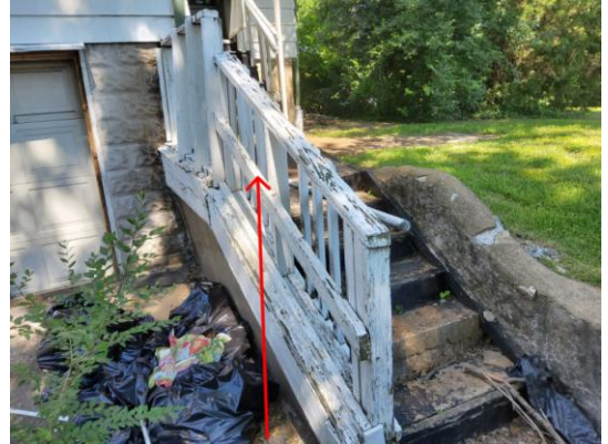
Photo 5: Railing Dilapidated .
