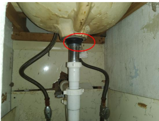
Photo 21: Pipe Leak.
