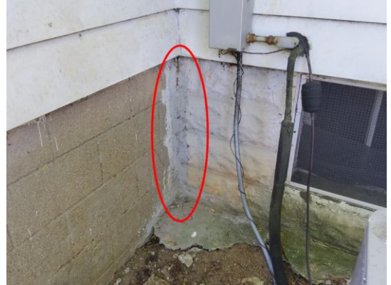
Photo 2: Prior Foundation Repairs.
