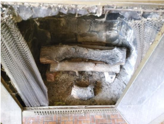
Photo 38: Inspect/Clean Fireplace Chimney.
