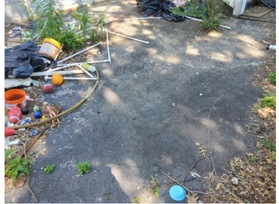
Photo 11: Driveway Seal / Minor Crack Repair.
