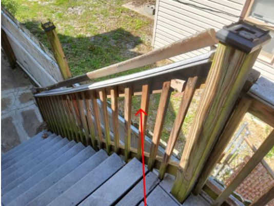
Photo 4: Railing Loose.
