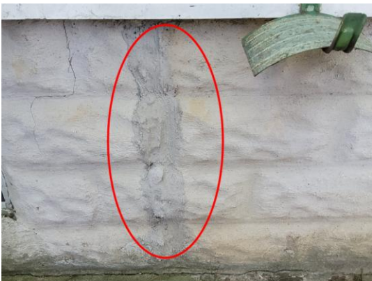
Photo 3: Prior Foundation Repairs.
