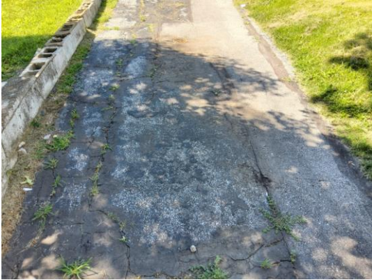
Photo 10: Driveway Seal / Minor Crack Repair.
