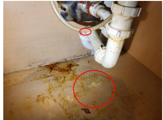
Photo 20: Pipe Leak.
