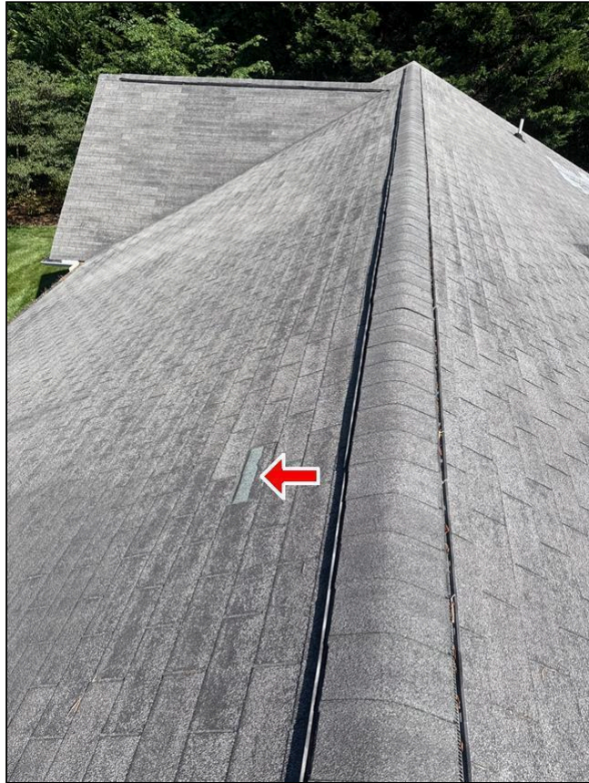
3.0 Item 2(Picture) Missing/damaged shingle tab
