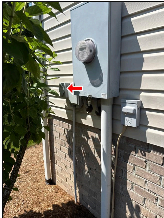
5.3 Item 2(Picture) Portable generator receptacle
