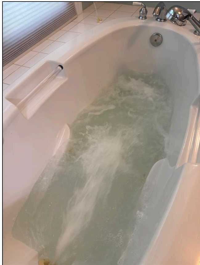
Jetted tub, in operation
