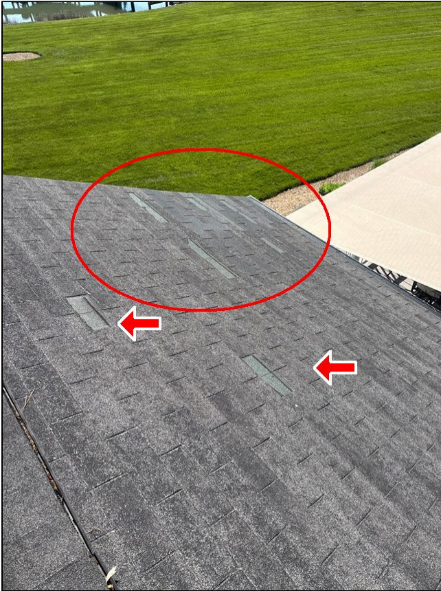
3.0 Item 1(Picture) Missing, damaged shingle tabs
