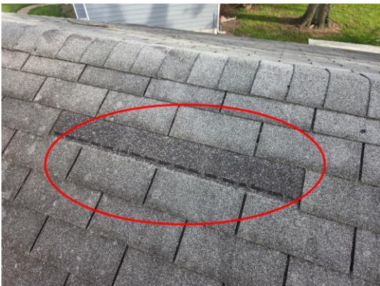
Photo 8: Minor Repairs Only.
