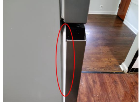
Photo 36: Door Gasket Poor.
