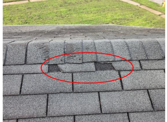
Photo 5: Minor Repairs Only.
