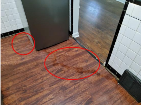
Photo 35: Refrigerator Leakage.
