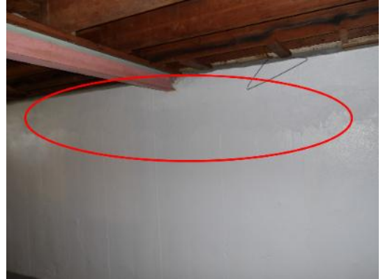
Photo 2: Prior Foundation Repairs.
