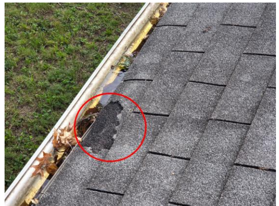
Photo 7: Minor Repairs Only.
