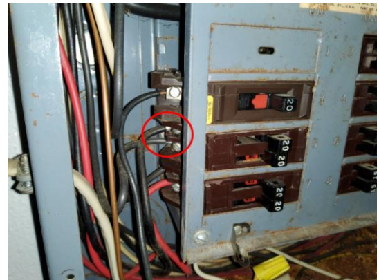
Photo 17: Aluminum Wiring.
