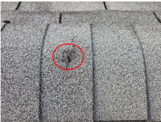
Photo 6: Minor Repairs Only.
