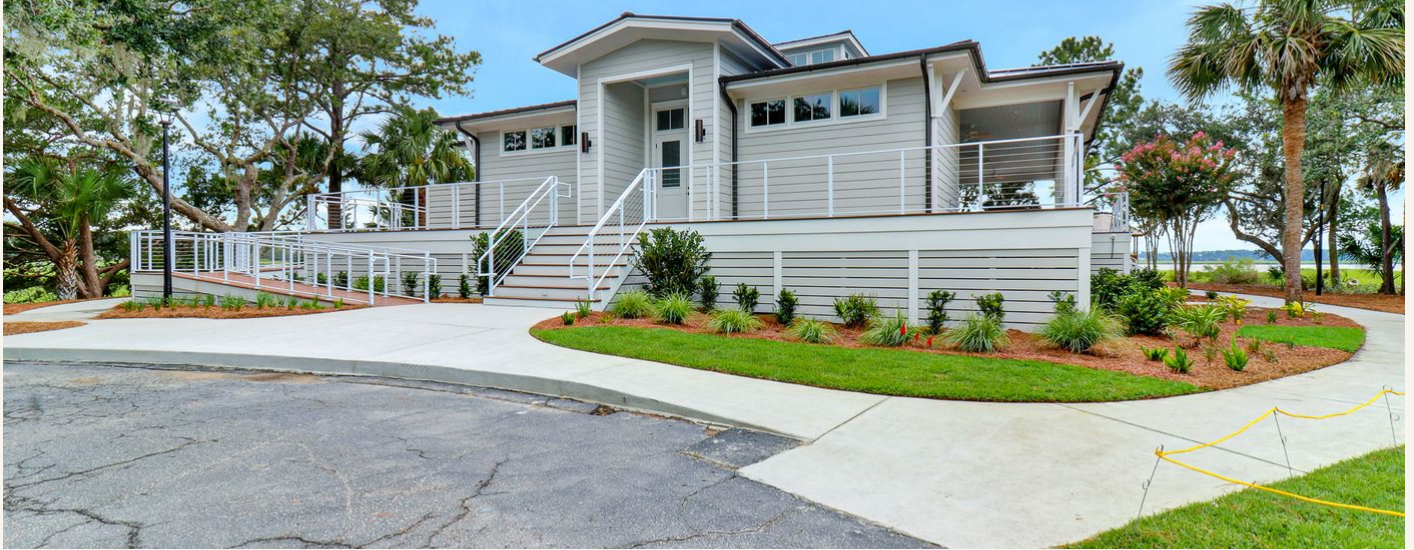
THE PAVILION AT COLLETON POINT LANDING, OVERLOOKING THE COLLETON RIVER
