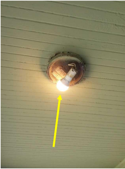
A light is missing its globe or cover and should be serviced.
