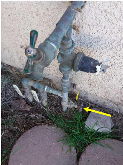
The main water shut-off valve is located at the right side of the house.
