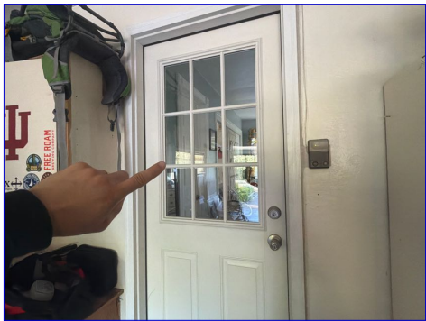
Window present at occupant door
