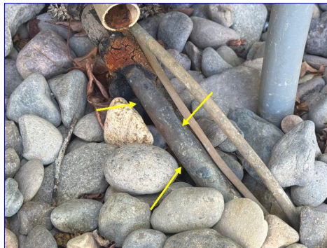
Missing insulation
