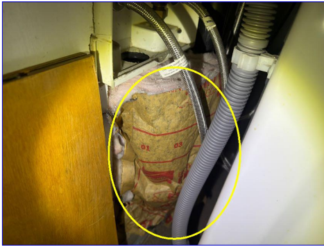
Exposed paper side of insulation
