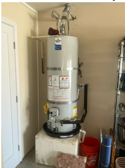
Hot water is provided by a 40 gallon gas water heater that is located in the garage.
