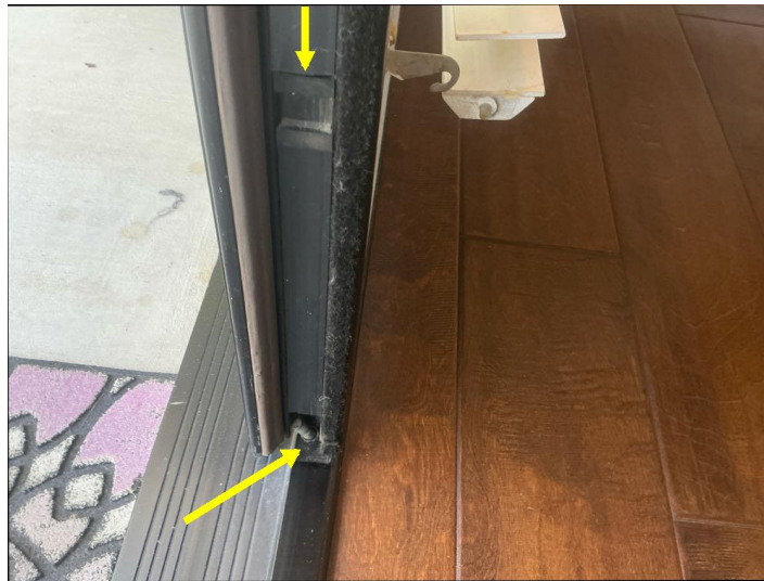
The stationary door closures serviced to be functional.
