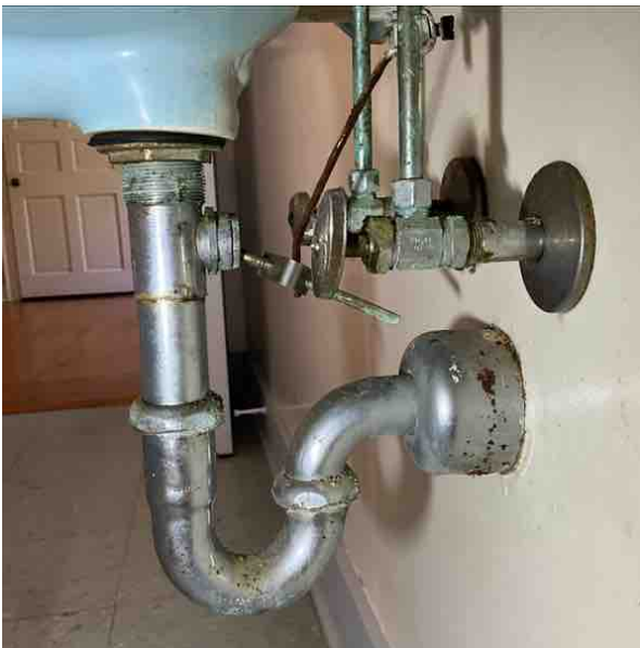
11.8.3 Drain lines are corroded and leaking, recommend replacement to limit leaks. (Kitchen)
