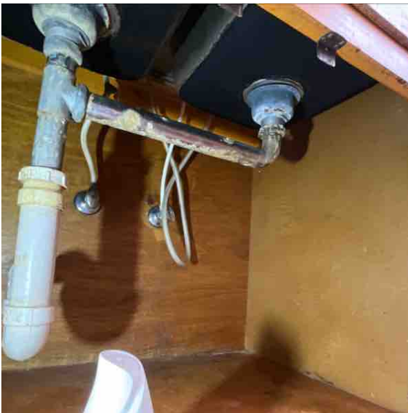
11.8.3 Drain lines are corroded and leaking, recommend replacement to limit leaks. (Kitchen)
