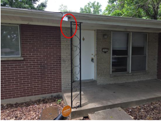
Photo 9: Downspout Missing .
