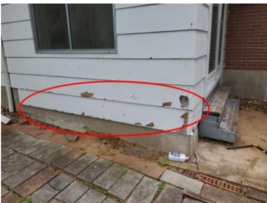
Photo 14: Wood Siding Paint.
