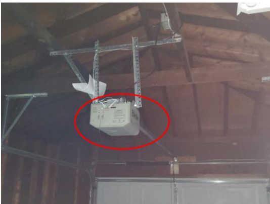
Photo 12: Operator Auto Reverse Defective, Laser OK.
