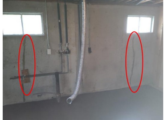
Photo 2: Prior Foundation Repairs.
