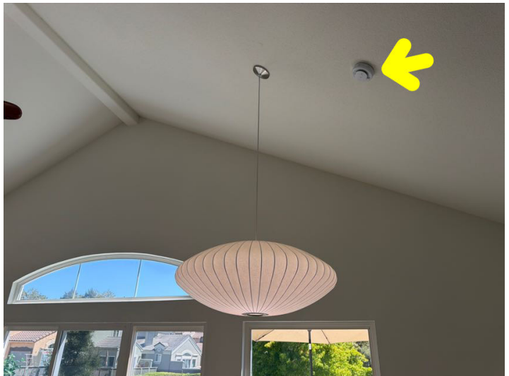
The smoke detector may not be in the location recommended by the manufacturer. We can elaborate but you may wish to verify this.
