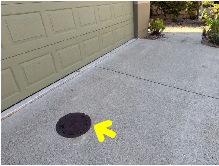
A clean-out is located at the front.
