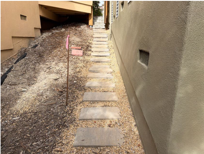
The railroad tie, paver, or natural stone steps are landscape components and would not conform to common standards requiring certain dimensions, handrails, guardrails, etcetera.
