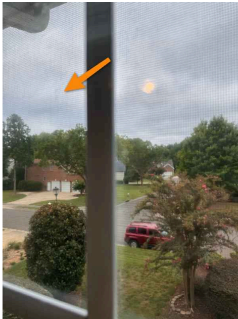
At least two sashes showed evidence of fogging
