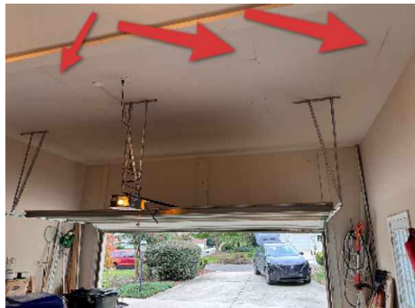
Garage door is causing ceiling drywall to crack and separate indicating poor support
