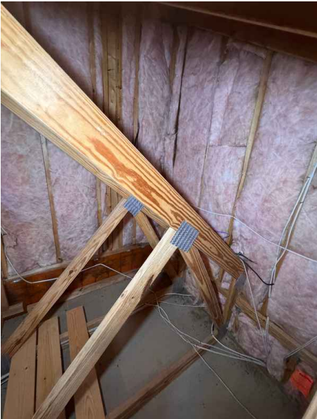
The corresponding area of the attic did not show any visible staining or damage
