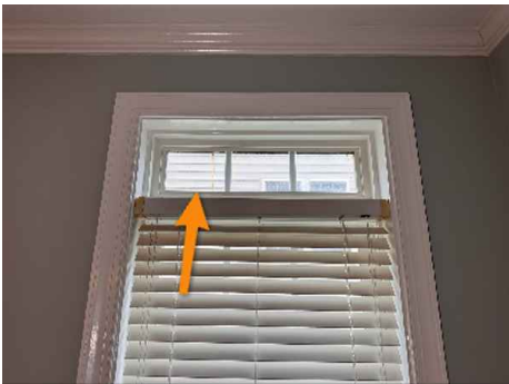
At least two sashes showed evidence of fogging
