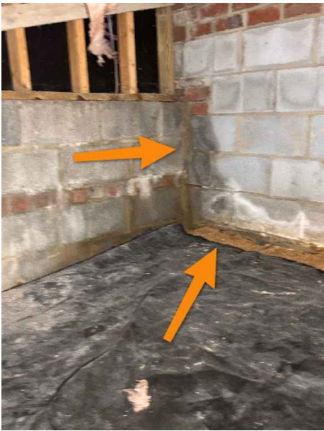
Evidence of water intrusion at the front center of the crawlspace
