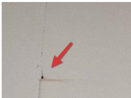
Garage door is causing ceiling drywall to crack and separate indicating poor support
