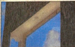
Window and door openings are pre-cut in the Structural Insulated Panels that make up this home near Ward.
