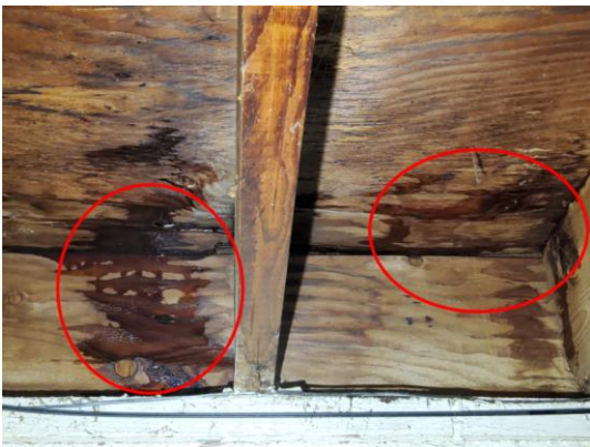
Photo 30: Pipe Leak.
