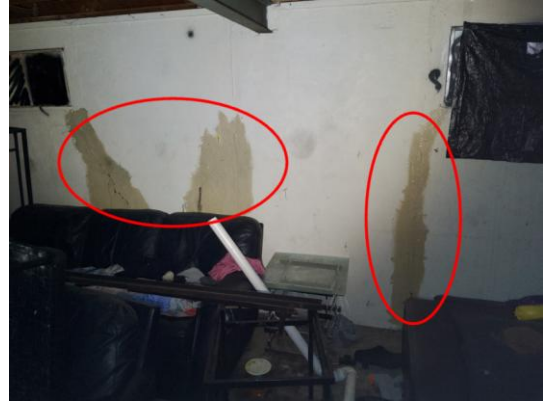
Photo 2: Prior Foundation Repairs.
