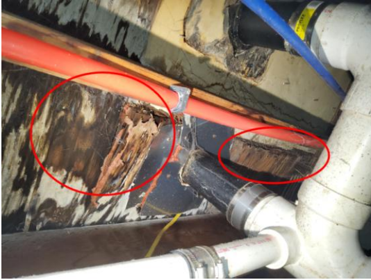
Photo 1: Damaged Subfloor.
