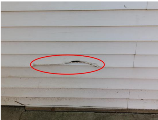
Photo 12: Siding Damaged.
